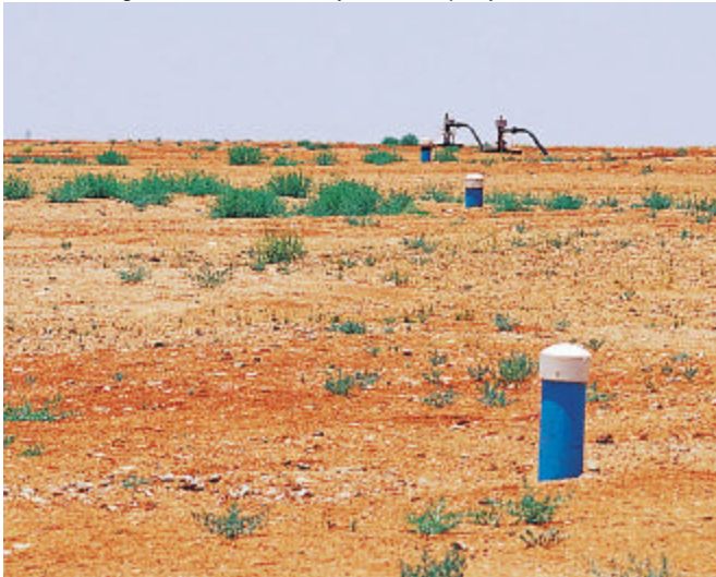
A monitoring well on the Beverley Mine Property
