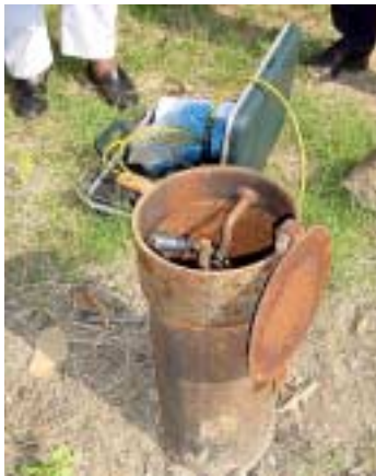
The well casing materials used at this site have begun to degrade showing heavy signs of rust.
